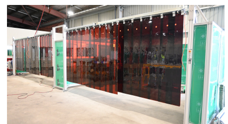
Welding curtains enclosing the U-6000 cell.
