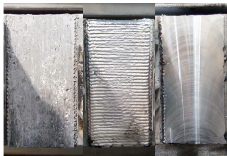
L-R: Before, Welded and After on a super structure repair.
