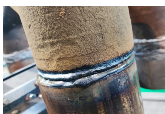
Finished weld result, between 7-9 passes, full penetration.
